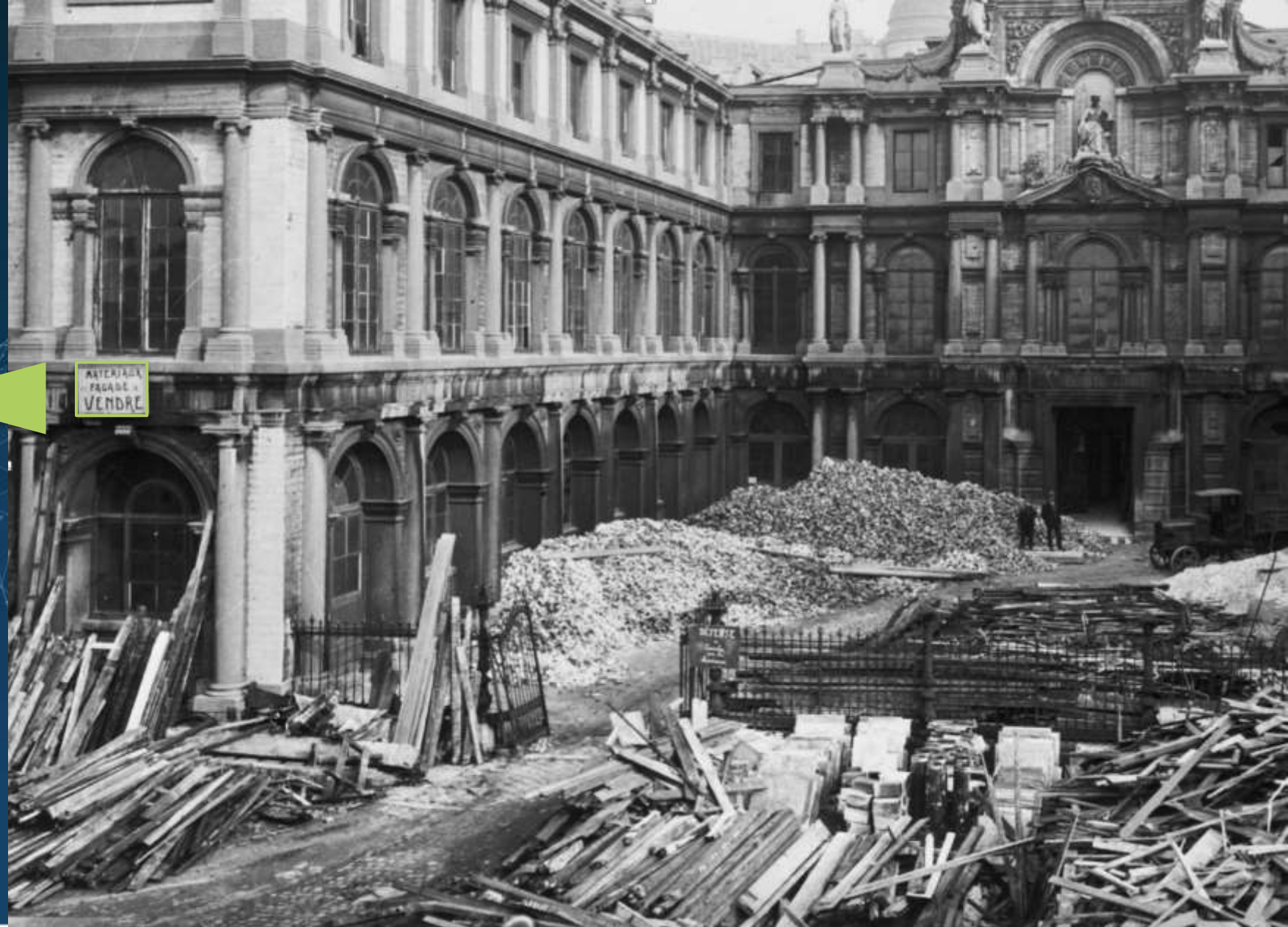
Brussels, 1928, Demolition of the Palais Granvelle, Building from 1550 KIK-IRP, cliché A105361
